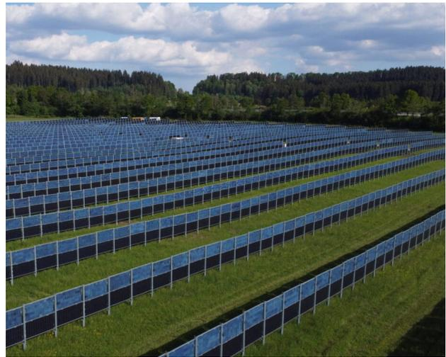
(b) Installation verticale. Source : <https://www.pv-magazine.com/2020/10/08/agricoltic-project-with-vertically-mounted-bifacial-panels-goes-online-in-germany/>
