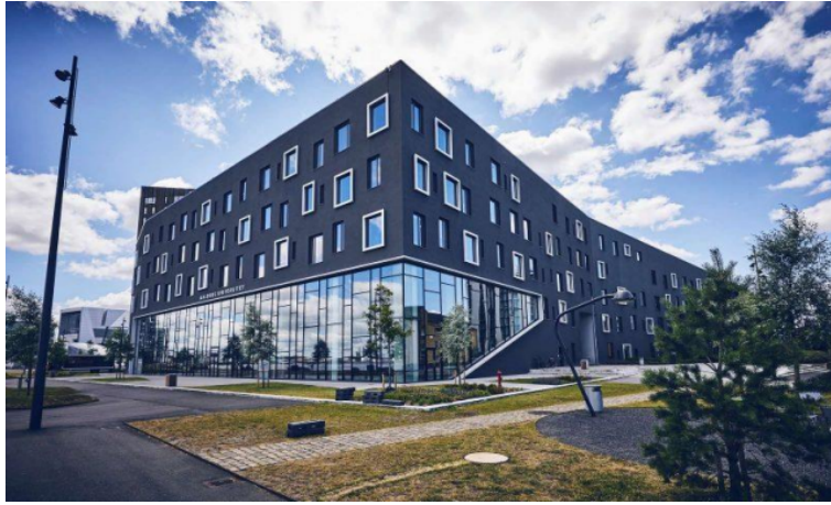
Figure 4.1: View of the building study case : CREATE - Rendsburggade 14, 9000 Aalborg, Denmark [2]
