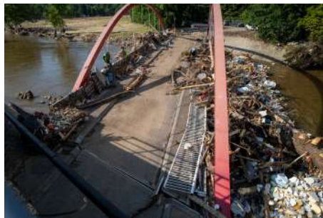
Figure 12: Clogged bridge in the Vesdre Valley.
