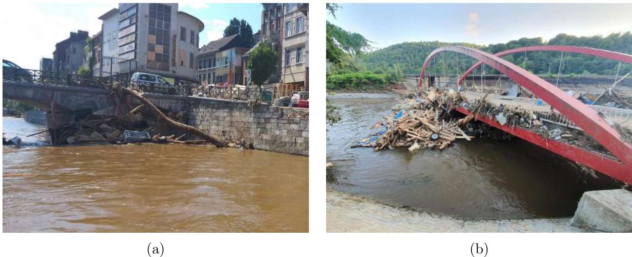
Figure 25: Large wood accumulations at bridges.
