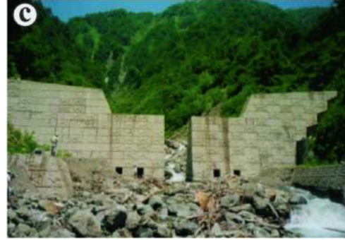
(b) Wang et al., 2022, fig.1(c), Slit-check dam in channel.
