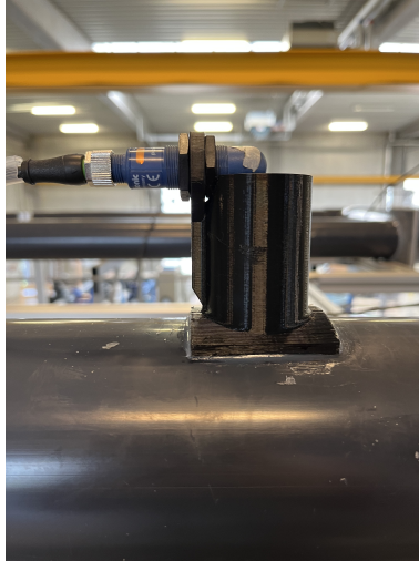
FIG. 15 Support that hold the pico+35/WK/I sensor above the pipe
