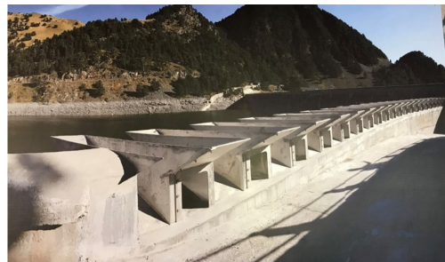
FIGURE 1.3: Oule dam - PKW (Defi12, accessed in June 2023).
