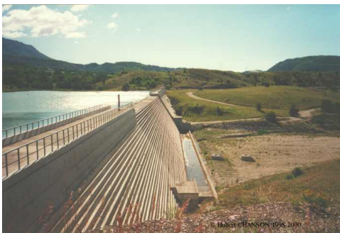
FIGURE 1.4: Riou dam (France) - stepped spillway (IAHR, accessed in June 2023).
