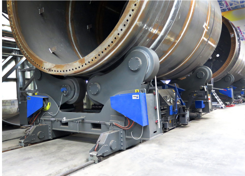
Figure 8: Roller welding beds are used for turning the structure for welding. Further, it helps to readjust the cans positioning in order to account for the slope of the conical cans. However, the steeper the angle the more the structure tends to fall off the rollers [16].
