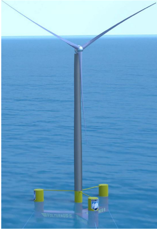
Figure 21: Key parameters and layout of the 15-MW reference floating offshore wind turbine [All+20]
