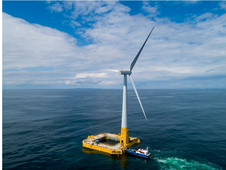
Figure 6: The Floatgen project using BW Ideol's 'Damping Pool' floating foundation [Ide23]
