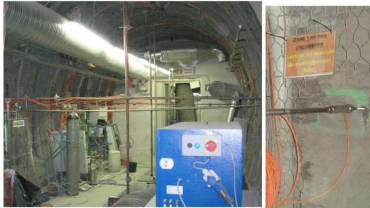
Figure 105: Convergence measuring devices in the gallery.
