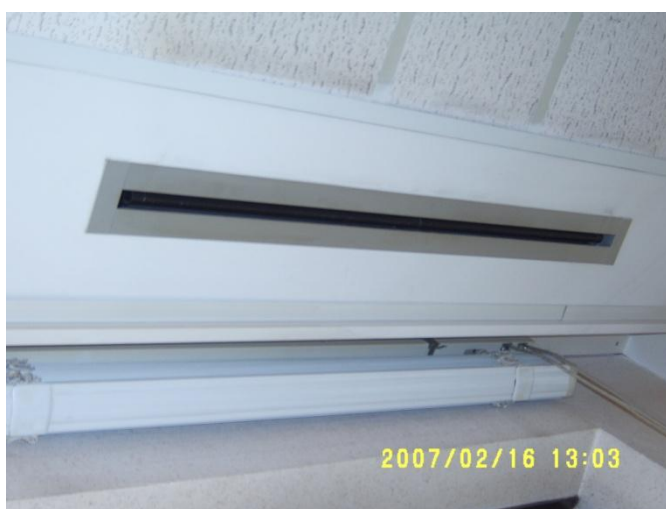
Figure 13 : Unité terminale VAV (Aparecida Silva et al. , 2008)
