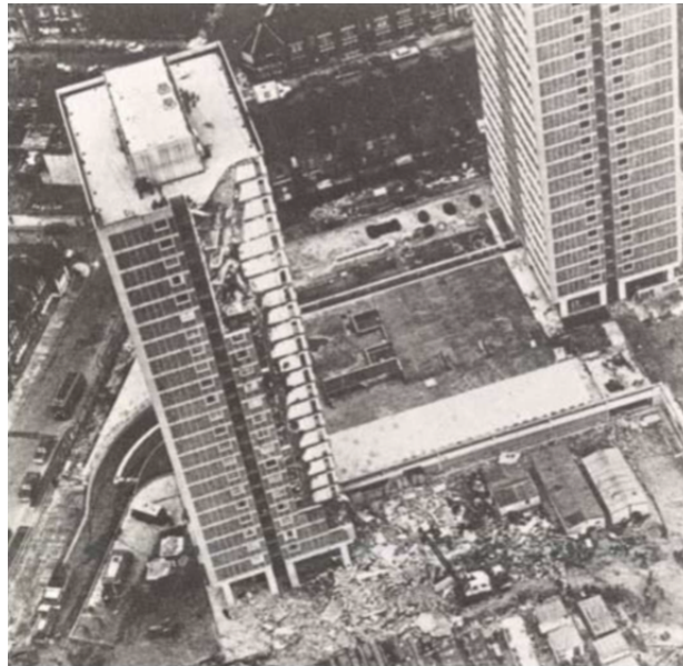
Figure I.1: The Ronan Point failure in 1968 [2]
