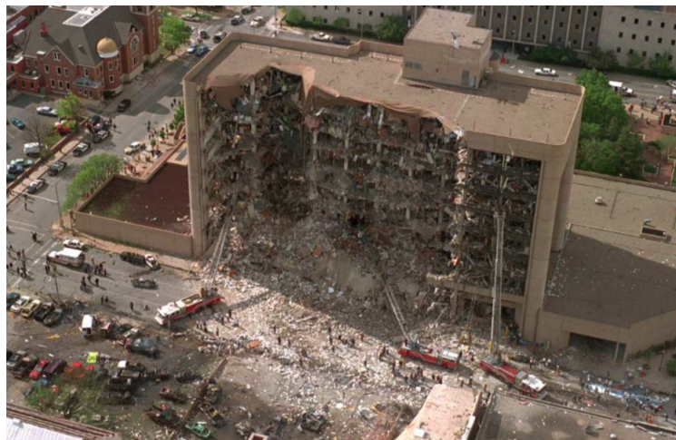
Figure I.3: The Murrah building failure in 1995 [2]
