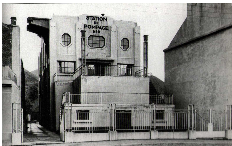
Fig.240 : La station de Jemeppe 09
