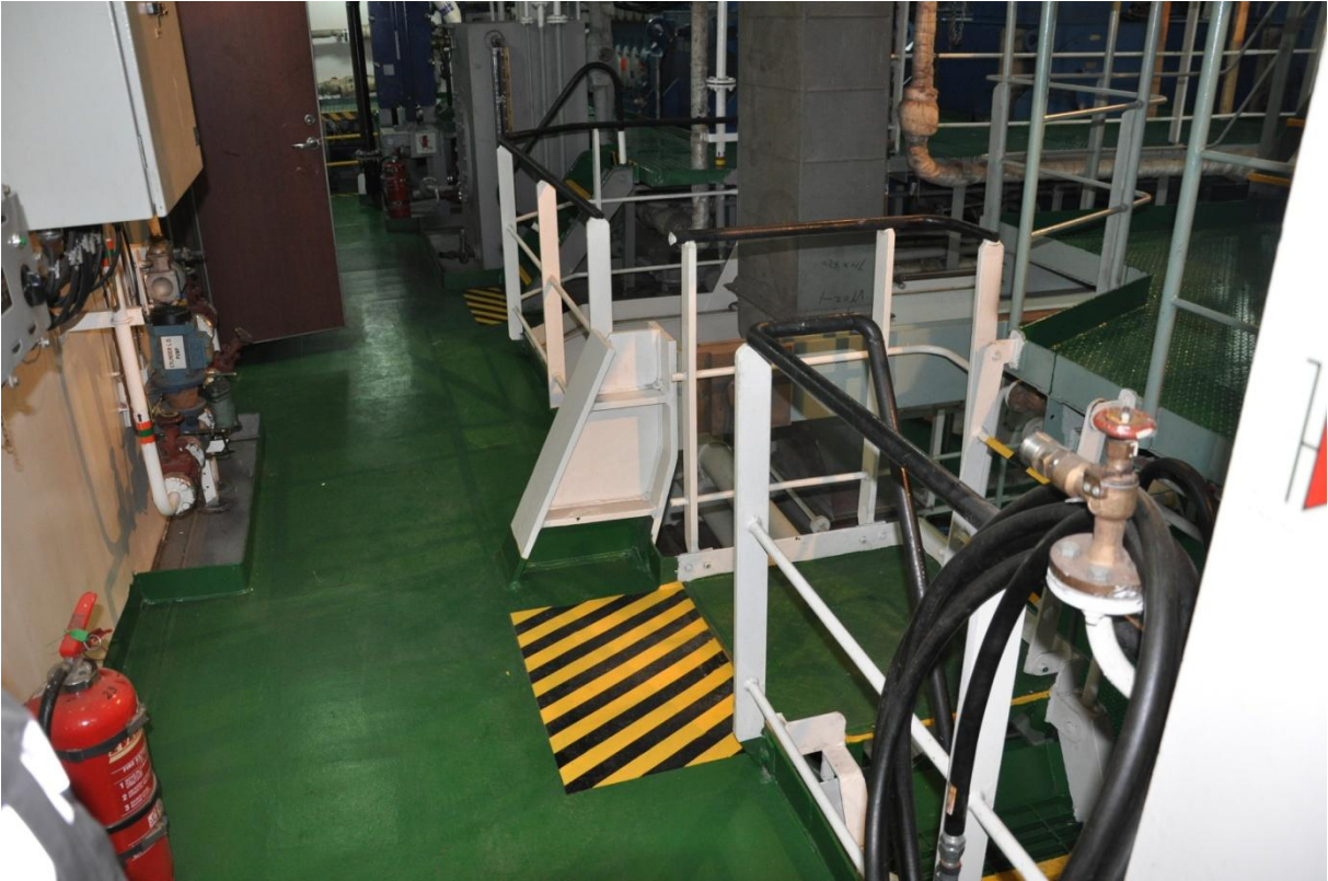
Figure A3.20 View on upper platform (driving end side)
