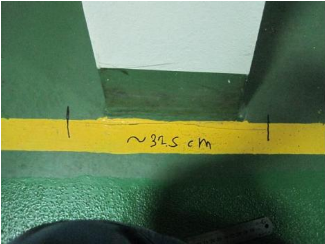
Figure 1.2 AFT side stay – crack at the bottom weld of the main support element.
