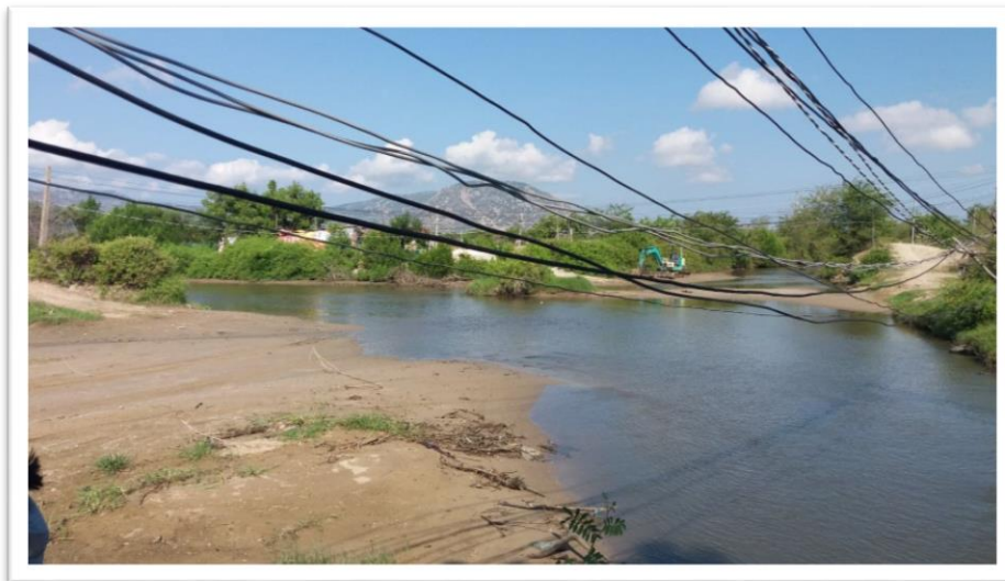
Figure 48: Irrigation canal in the Phuong Hai commune
