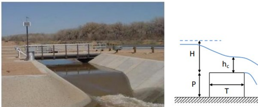
Figure 2.3: Flow over a broad-crested weir
