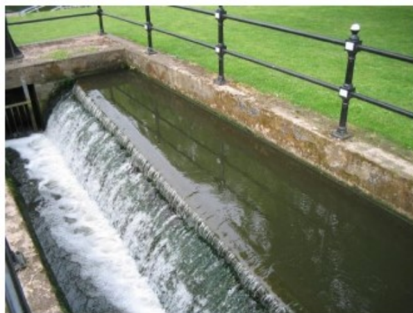
Figure 2.5: Flow over a side weir
