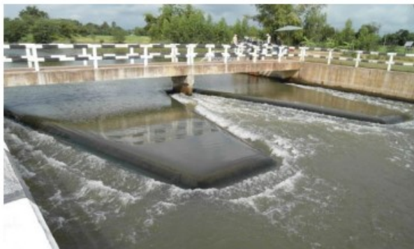
Figure 2.6: Flow over a labyrinth weir
